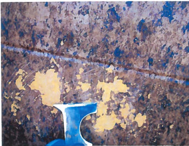
Detail of Carboline panel (P-10) 510 SG/Fiber Reinforced PolyBrid 705.
