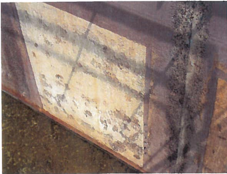
Overview of Saureisen panel (P-12) F-121 resurfacing material and 210 Glaze topcoat.
