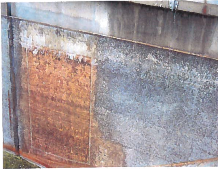
Overview of Carboline 510 SG resurfacing material and PolyBrid 705 panel (P-16).
